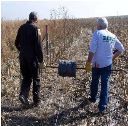
USGS workers install a fence on CRP land. From http://biology.usgs.gov/cro/ScienceInYourState/Montana/MT-brd.htm
